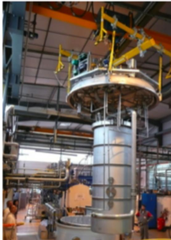
*Cryostat (before floor construction)*
